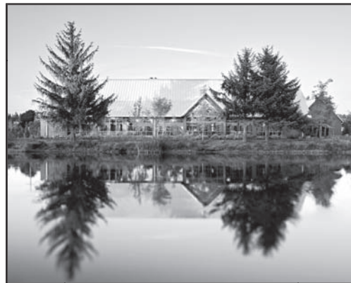
Estacada Public Library at dusk viewed from the future Wade Creek City Park.
